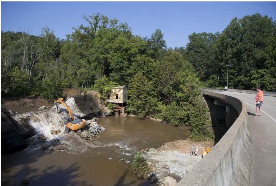
Figure 2.3.1 – Removal of the Power Dam. This has created an ongoing concern about water quality in the Pigg River.
